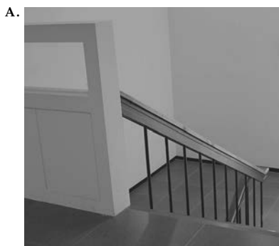
FIGURE 1.5. Accidental Affordances Can Become Strong Signifiers. This wall, at the Industrial Design department of KAIST, in Korea, provides an anti-affordance, preventing people from falling down the stair shaft. Its top is flat, an accidental by-product of the design. But flat surfaces afford support, and as soon as one person discovers it can be used to dispose of empty drink containers, the discarded container becomes a signifier, telling others that it is permissible to discard their items there. (Photographs by the author.)
